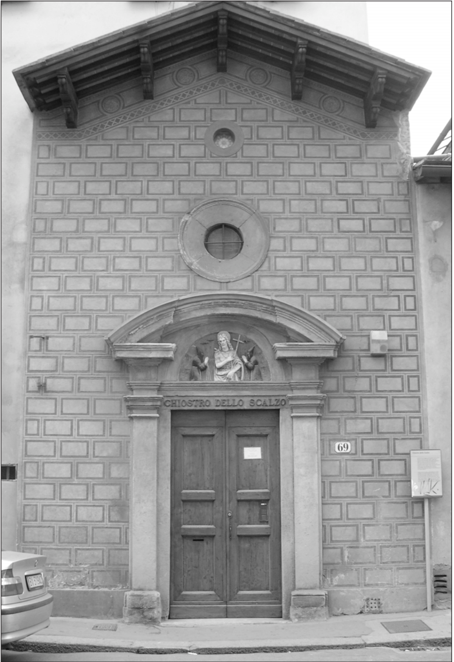
Fig. 1. Entrance to the Chiostro dello Scalzo, Via Cavour, Florence (Photo: author)
